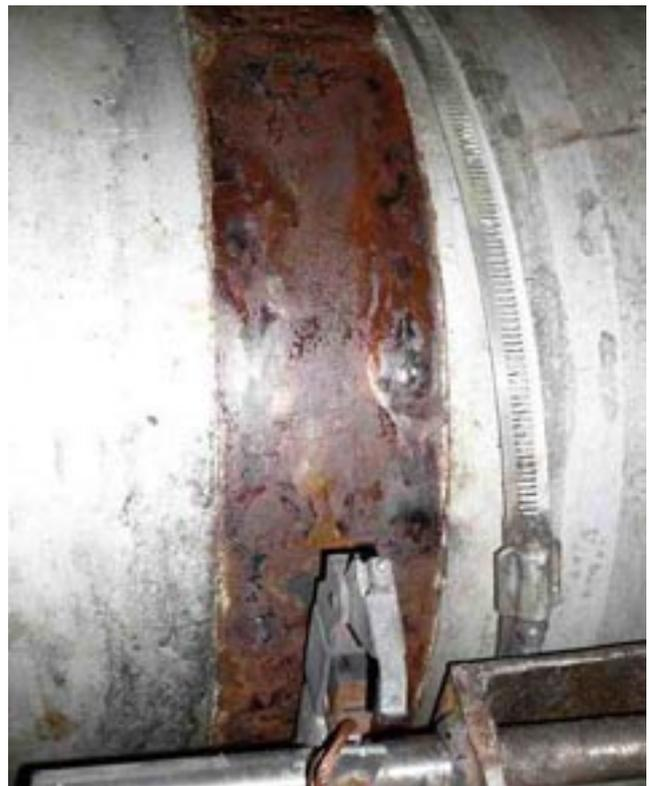
*Corrosion hiding behind the slip ring*
